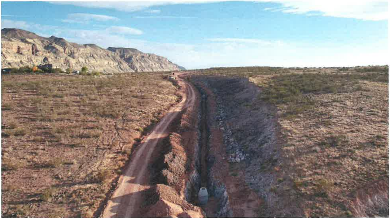
Figure 4: Main sewer line trench in Copper Rock Parkway to North Slope.
