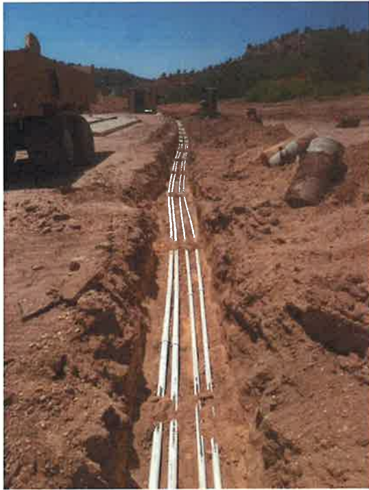
Figure 1: Open trench of supply and return treated effluent lines
