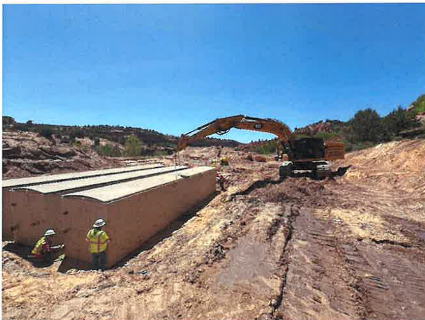
Figure 2: Effluent treatment units being set by ACAD crew.
