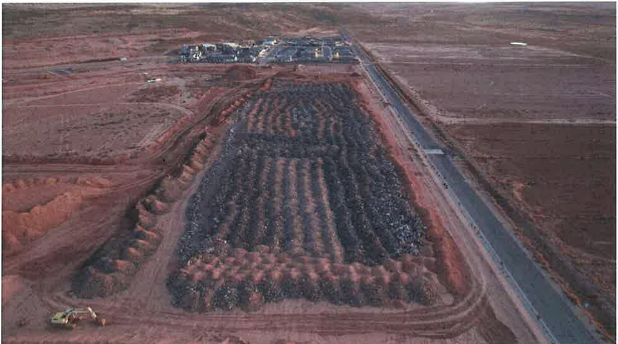
Figure 5: Material stockpile, conditioning, and rework for North Slope lots and roadways.
