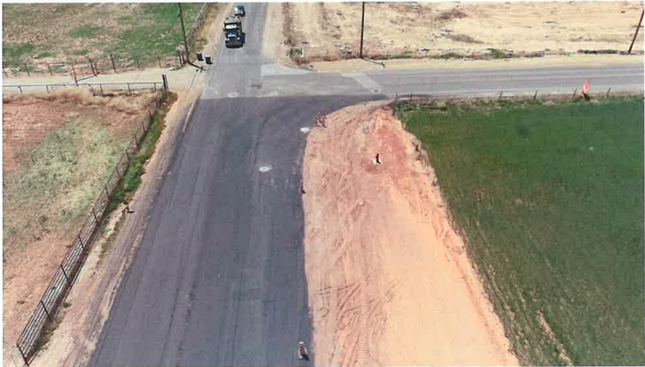
Figure 3: Aerial view of 1100 W roadway in Hurricane, UT after asphalt pavement and before striping. View shows new pavement tie-in starting at 3000 S along with new valve collars, and a new fire hydrant.
