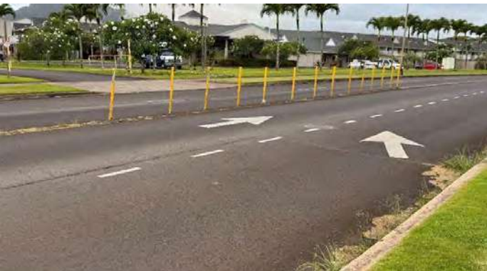
Flexible delineator with rubber curb
