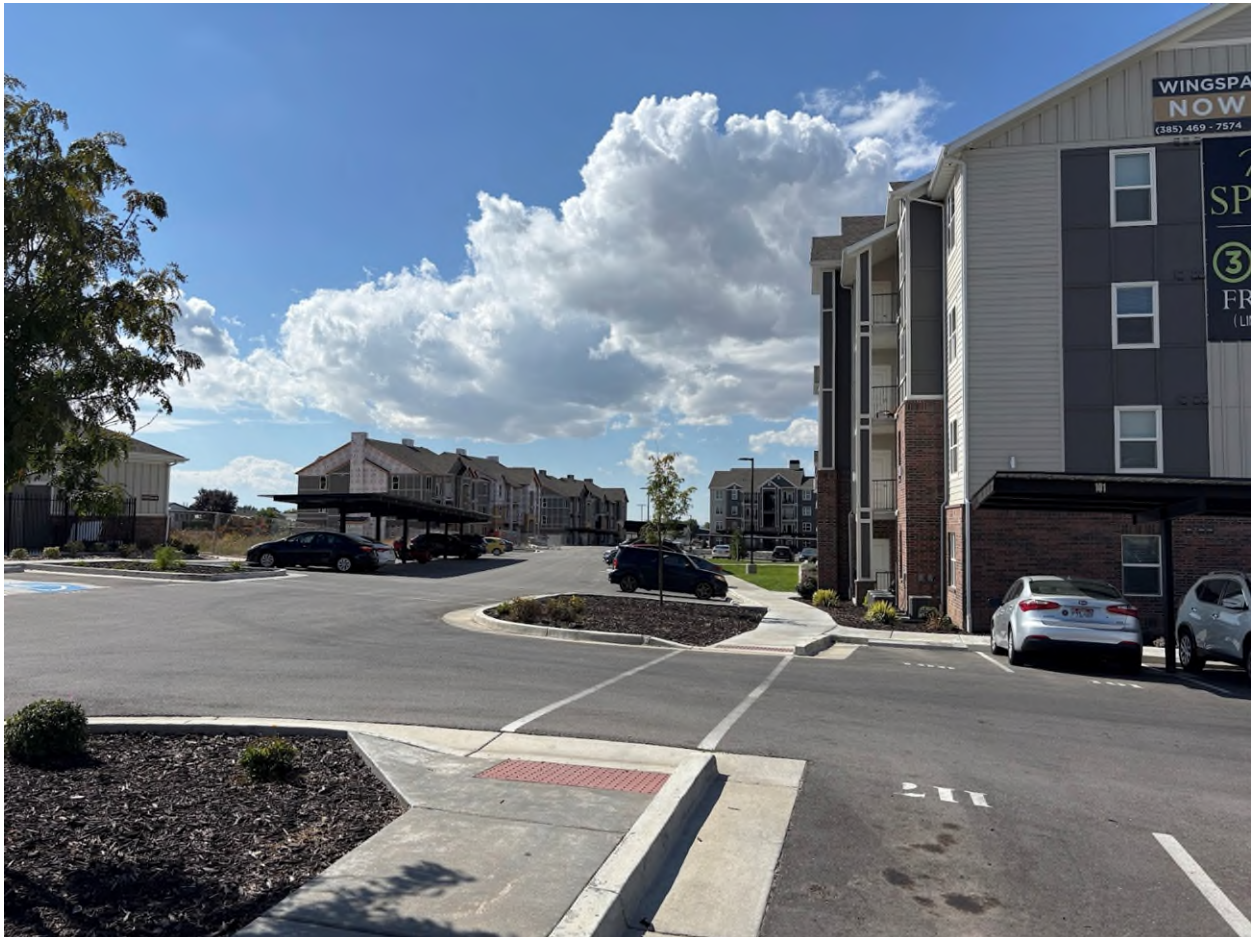
Image 2-Wingspan Apartments within the R-3 Zone
