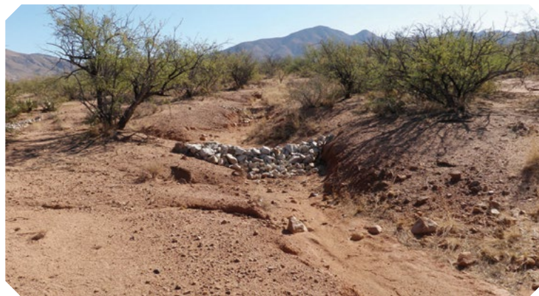
Check Dam, Erosion Control Research Program
