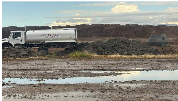
Onsite Material Stockpile
