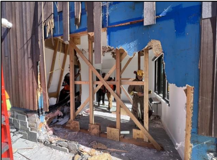
Deer Valley East Village structure shoring
