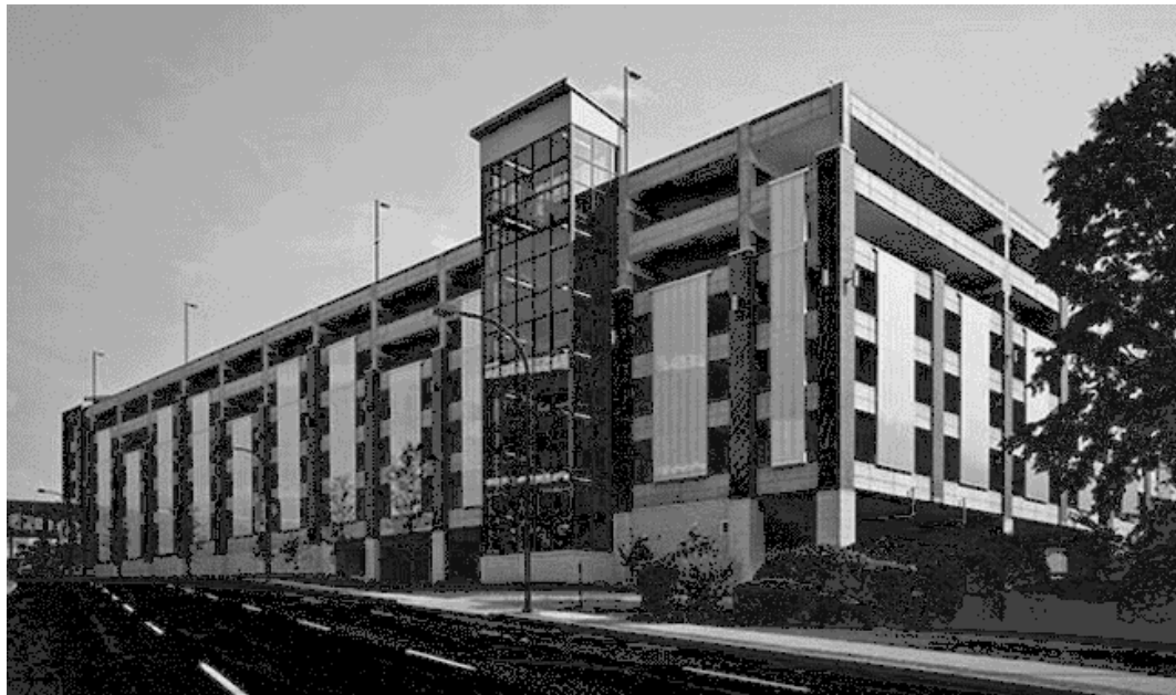
FIGURE I - EXAMPLE PARKING GARAGE STRUCTURES
