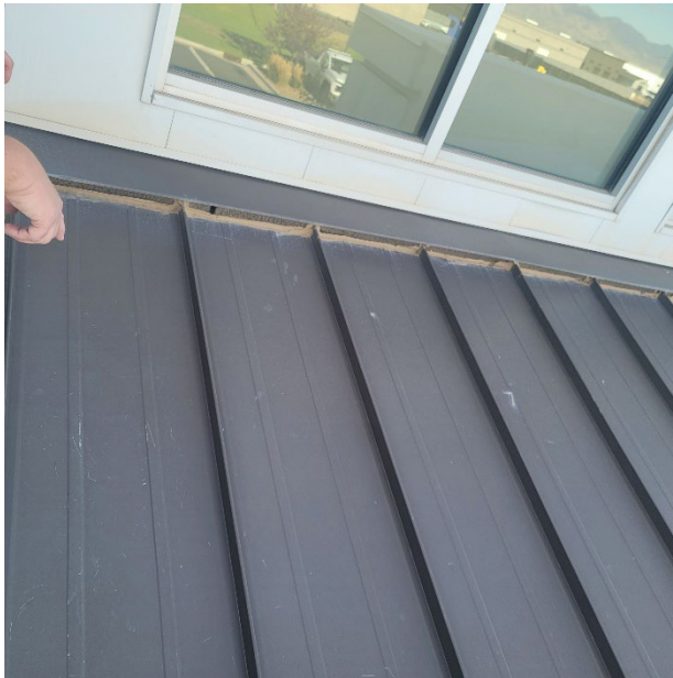
Figures 5 & 6 - Water intrusion at roof to wall connection and metal roof over membrane roof at parapet walls on west side of building.
