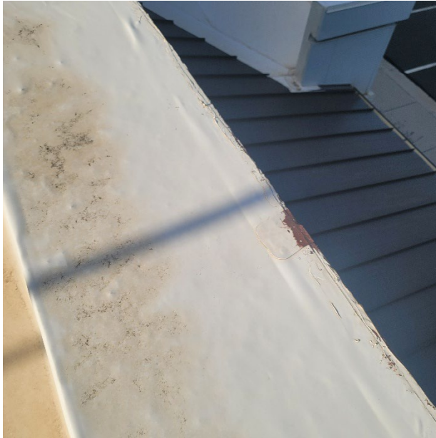
Figures 1 & 2 - Membrane roof fastened to the top of drip metal continues to leak.
