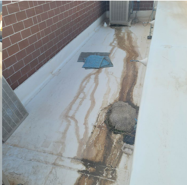
Figures 1 & 2 - Membrane roof fastened to the top of drip metal continues to leak.
