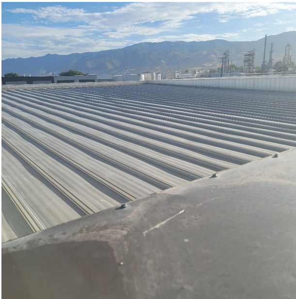
Figures 7 & 8 - Galvanized metal roofs routinely leak at top parapet walls, side parapet walls, and at the gutter adjoining the bottom parapet wall.
