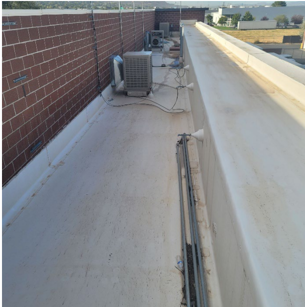
Figures 3 & 4 - Multiple patches and leaks in membrane roof materials.
