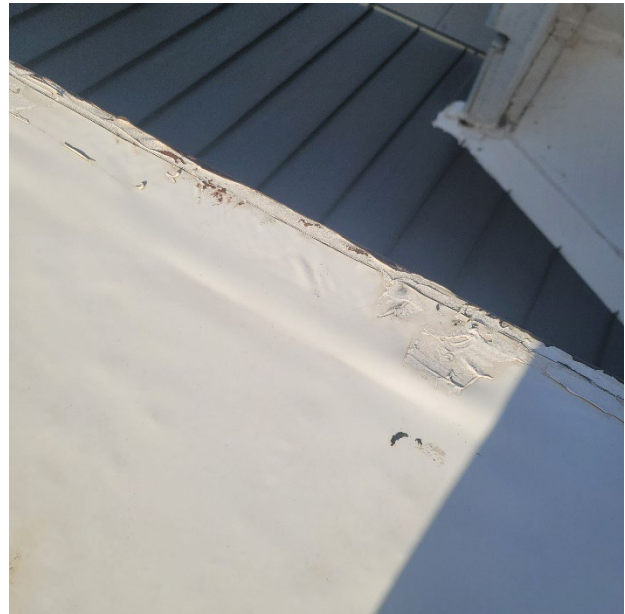
Figures 1 & 2 - Membrane roof fastened to the top of drip metal continues to leak.
