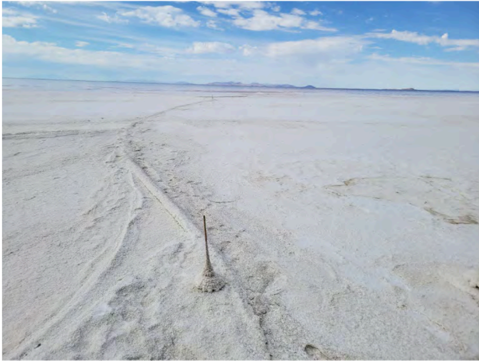
Centerline staking, looking West.
