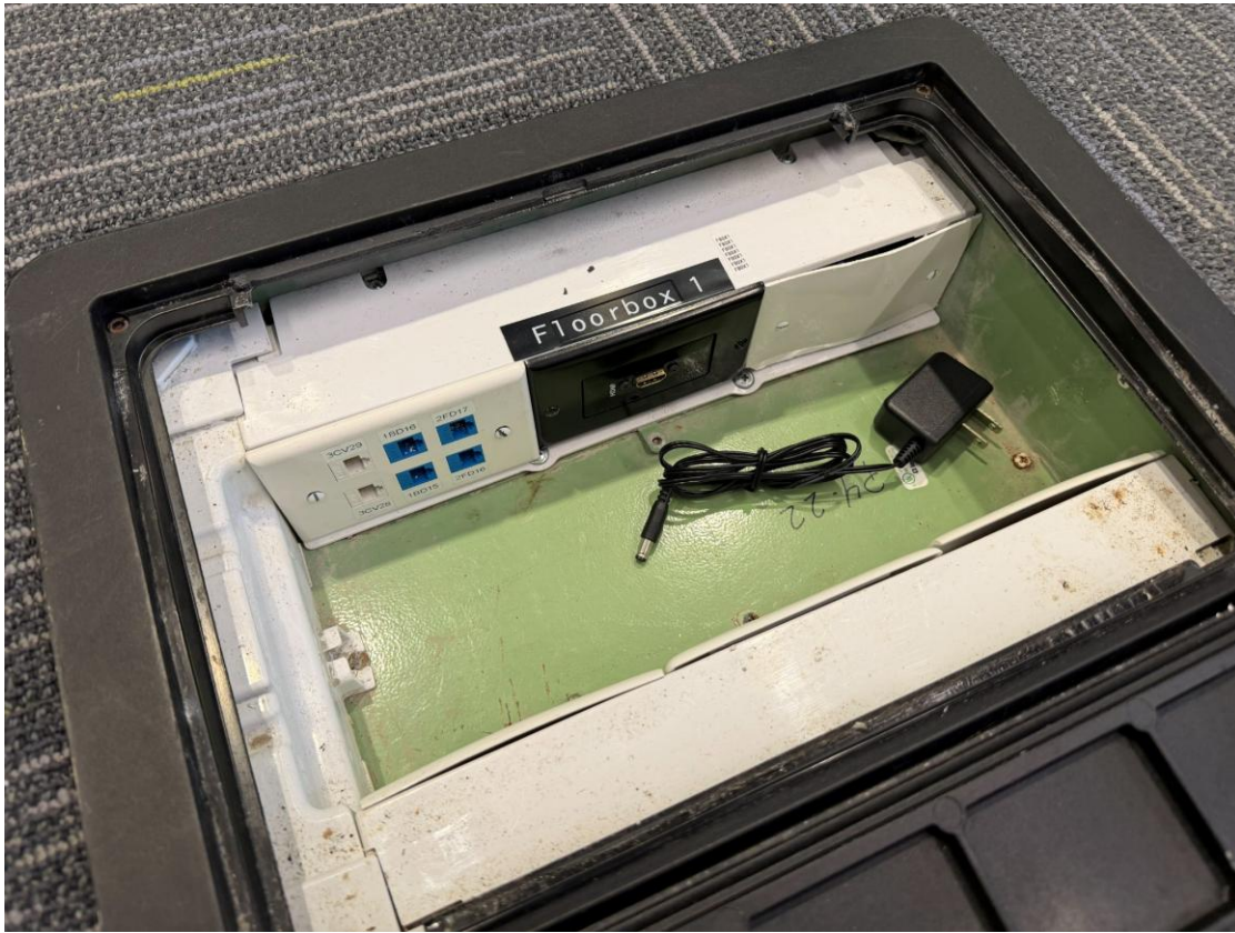
Figure 13. Police EOC – EOC East-Wall Media/Press Connection – Existing network jack and conduit for use with the required media/press feed.
