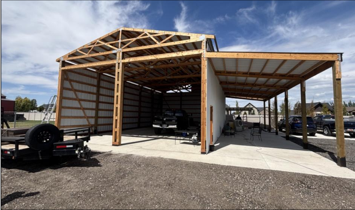
Photograph 2: Shop Constriction In-Progress 8/1/2026
