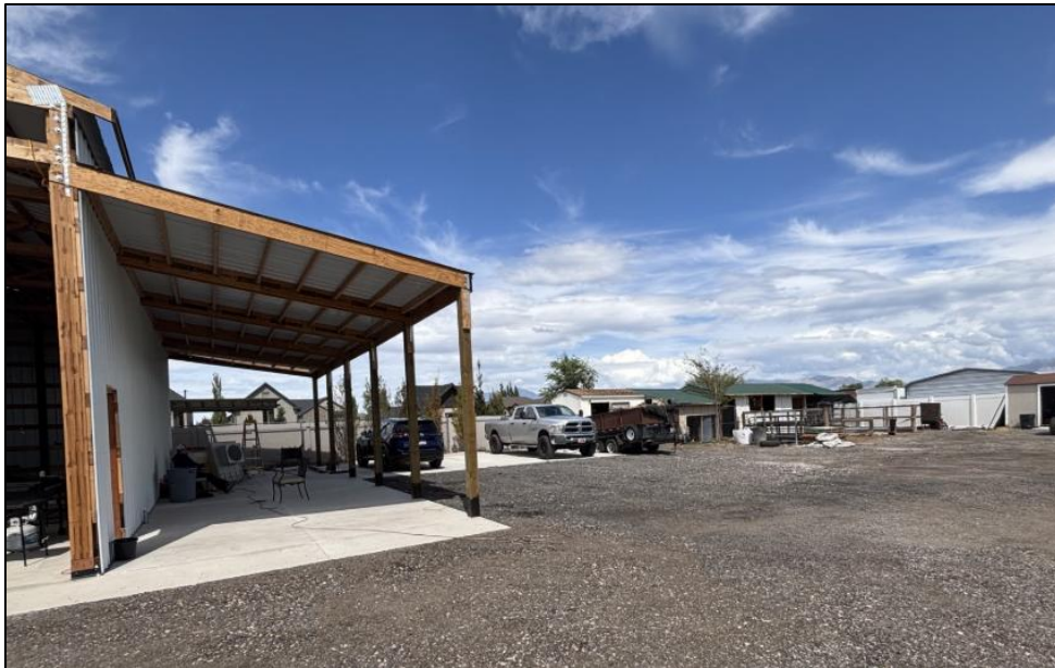
Photograph 1: Employee Parking Pad and Milled Asphalt Driving Surface 8/1/2026
