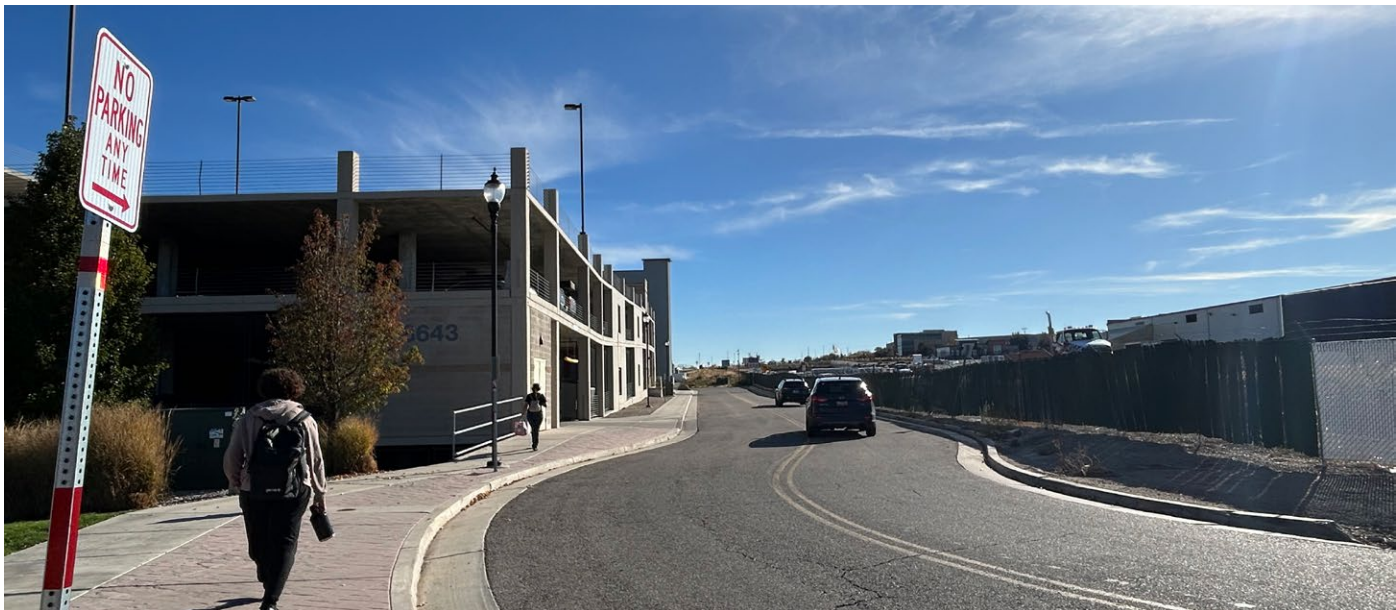
Jordan Valley Station: UTA Parking Structure
