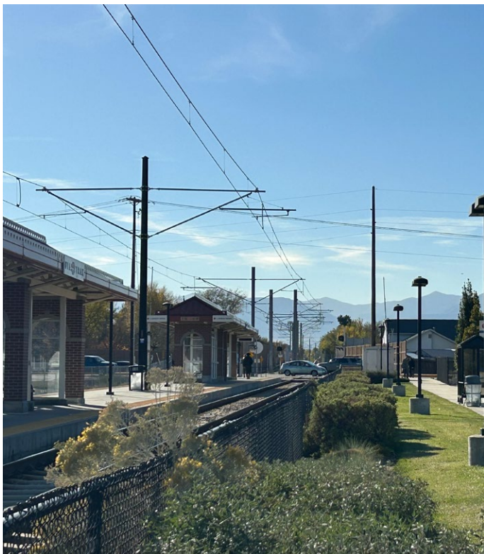
Sugar Factory Rd. Station Platform, Source: Design Workshop
