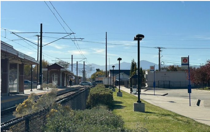
Sugar Factory Rd. Station: UTA Parking Lot
