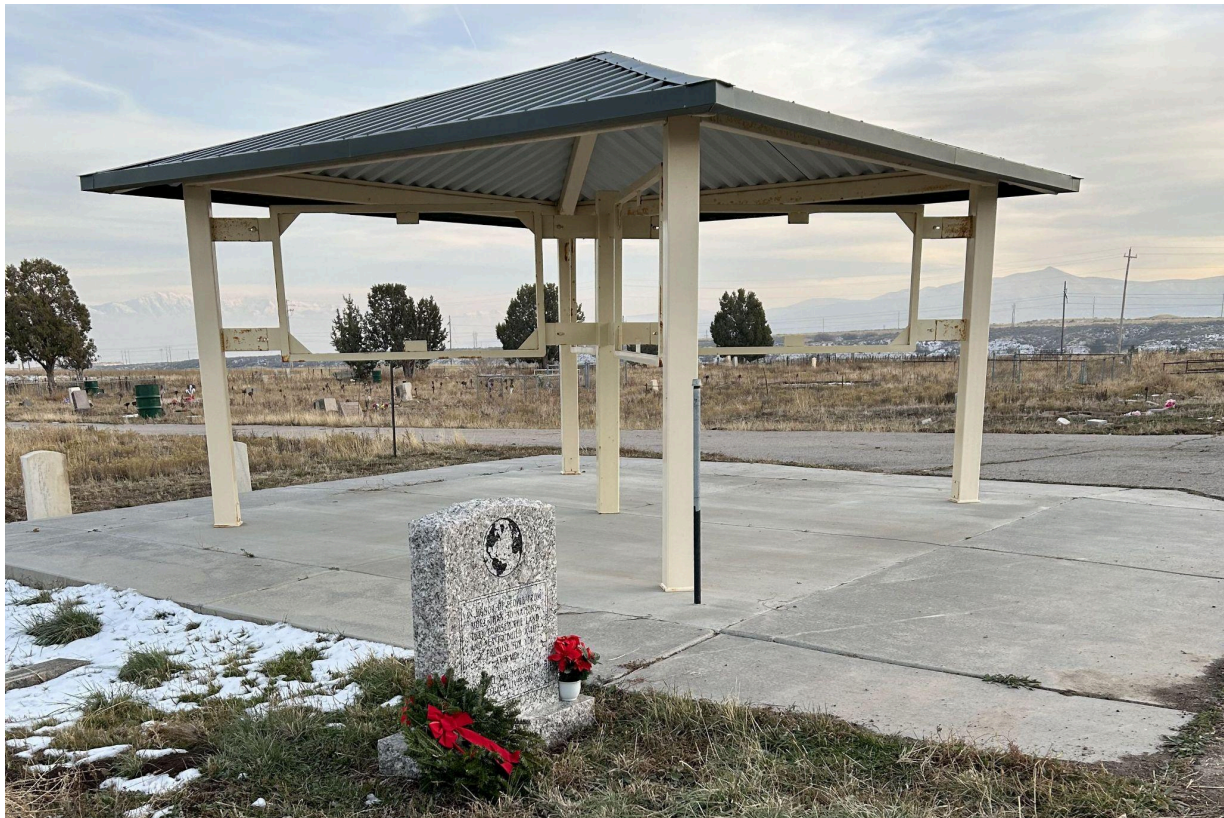
Photograph: Existing Memorial Pavilion
