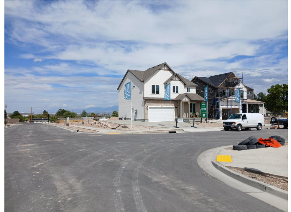
Subdivision utility install construction complete and current status
