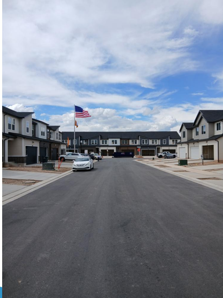
Phase 1 development progress
