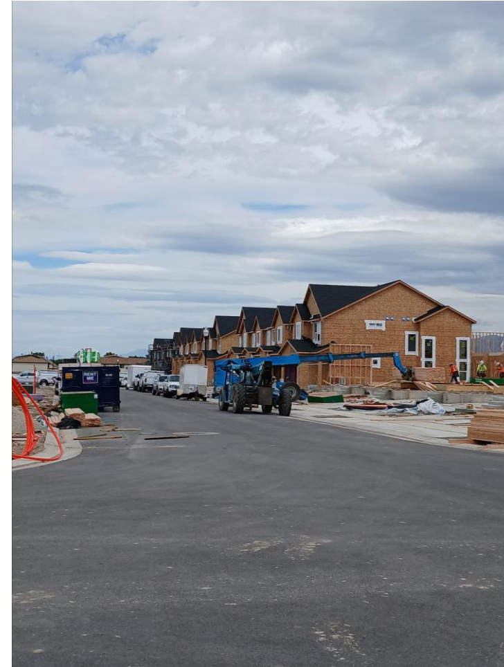
Phase 3 development progress
