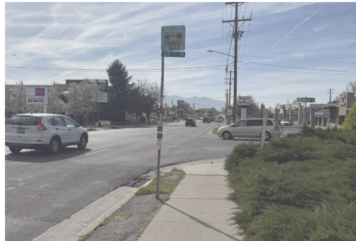
Unimproved transit stop along 3300 South
