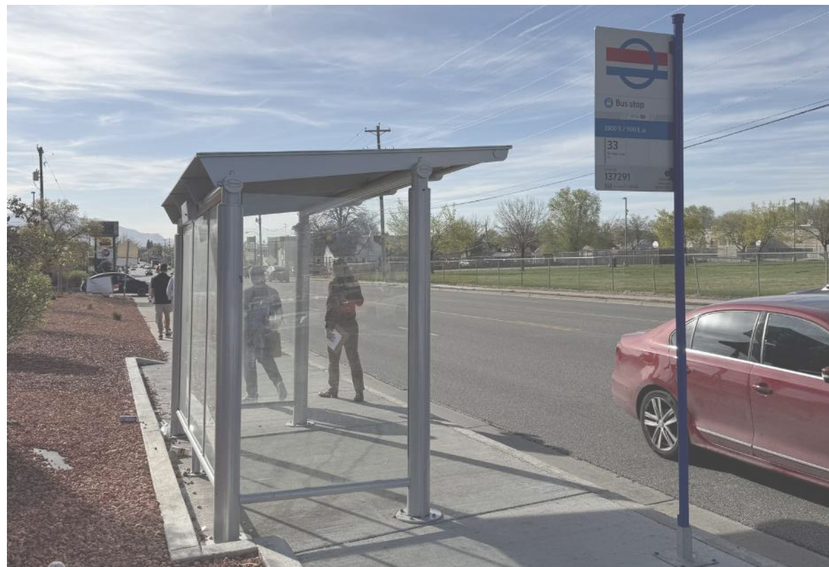
Improved transit stop along 3300 South
