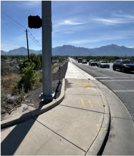
LOOKING EAST ALONG 5400 S AT RECENTLY COMPLETED NORTH SIDE SIDEWALKS.
