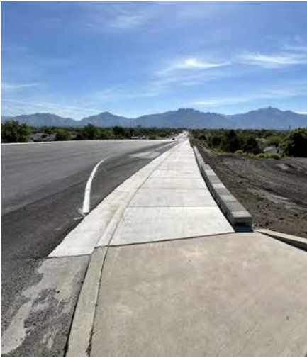
LOOKING EAST ALONG 5400 S AT RECENTLY COMPLETED SOUTH SIDE SIDEWALKS.
