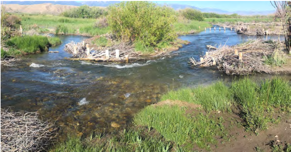
LEMHI RIVER, 1.5 YEARS AFTER CONSTRUCTION OF MULTI-THREADED CHANNEL NETWORK USING VARIOUS BANK AND INSTREAM STRUCTURES TO SPLIT FLOW INTO MANY, SHORT, NARROW SIDE CHANNELS.
