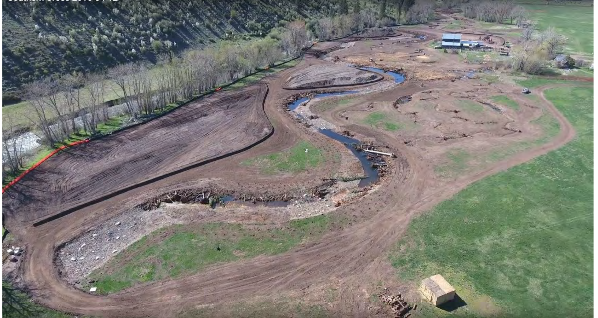
IN-PROGRESS CONSTRUCTION ON THE CHANNEL REALIGNMENT OF CATHERINE CREEK IN OREGON.
