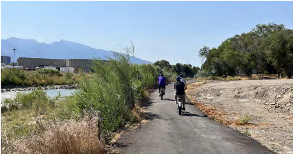
GROUND LEVEL VIEW OF JORDAN RIVER PARK TRAIL WITH MURRAY CITY'S PUBLIC WORKS FACILITY ACROSS THE RIVER IN THE BACKGROUND.
