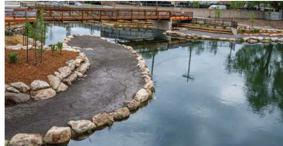
EXISTING WATER GET-DOWN AT THREE CREEKS CONFLUENCE PARK AT 1300 SOUTH AND 900 WEST
