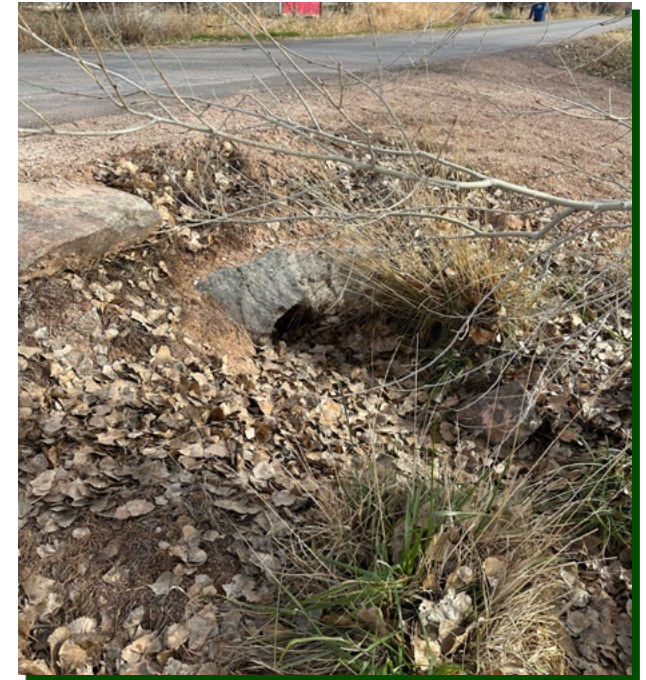
South Pocket Park Culvert
