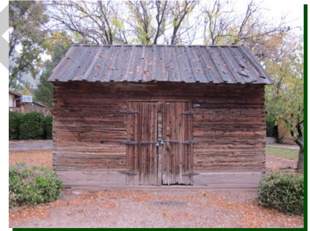
Historic Town Hall Jail
