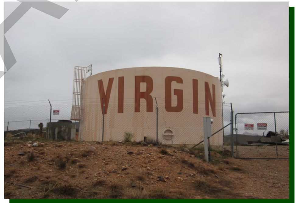
Virgin Main Water Tank
