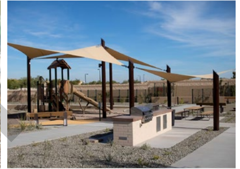
Shade structures over playground
