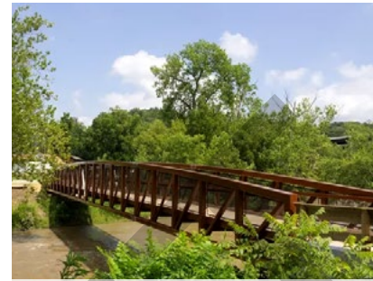
Pedestrian bridge over river
