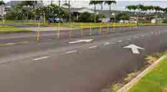
Flexible delineator with rubber curb
