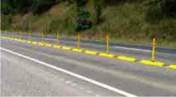
Flexible delineator with rubber curb
