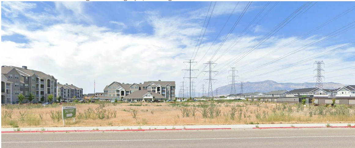
Image 5: Photograph, Existing conditions with RMP Power Lines
