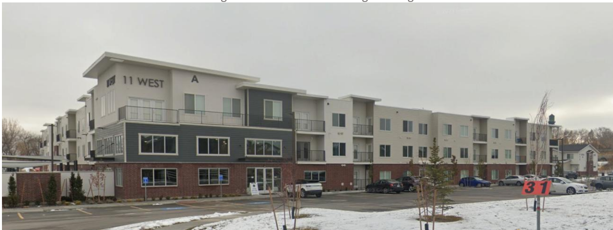
Image 5: Street View of Existing Building
