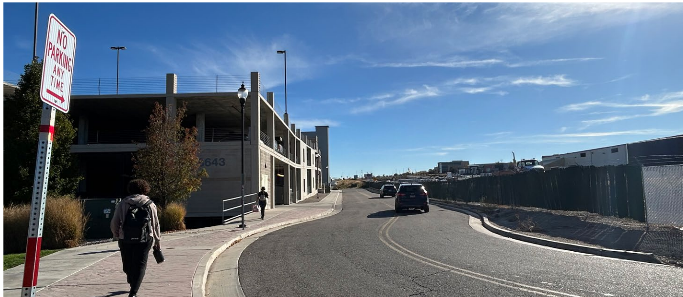
Jordan Valley Station: UTA Parking Structure
