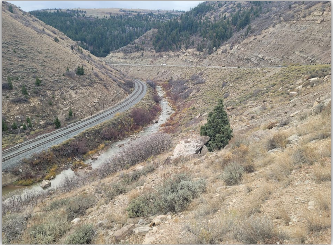
Image 3: View of Price Canyon with the Price River and existing infrastructure, including Highway 6, the UPRR, and overhead powerlines. Photo taken at the western end of the Project Area on October 2025, facing south (WESTERN-ENVIRO Resources, Inc. 2026).
