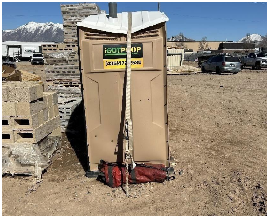
Figure 28: Photo showing portable toilet secured with tie-down straps
