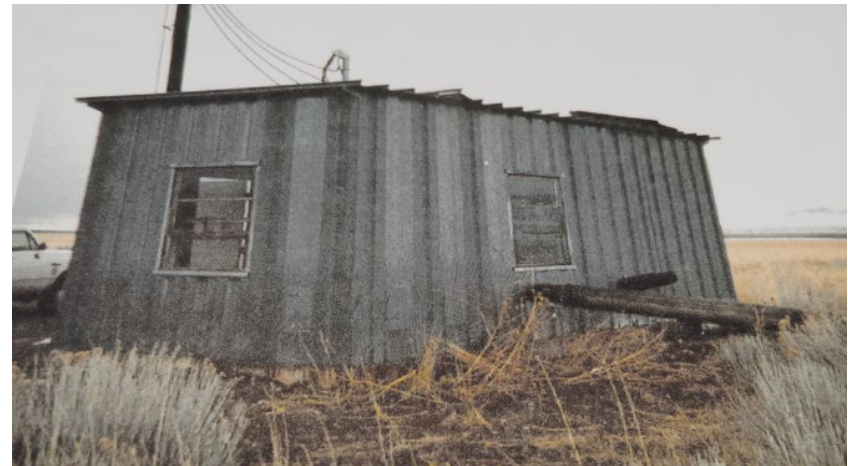
Old Quichapa Well #3 Building (built in ~1967, photo in 1996)
