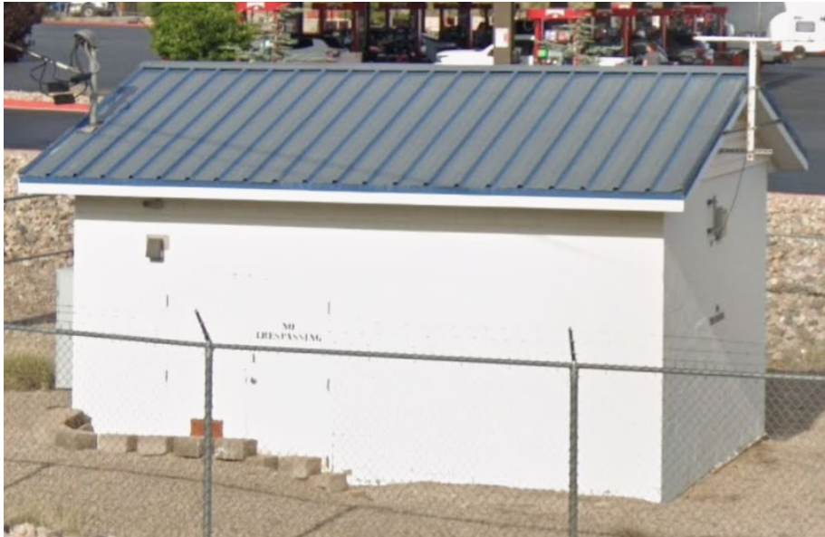
Square Mountain Pump Station (built in 1994)
