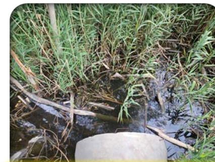
Tuscany Det Pond Outfall Inspection
