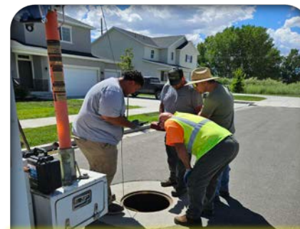
Team Televising in Manhole
