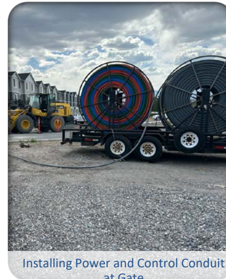
Installing New Conduit for Gate Power and Controls
