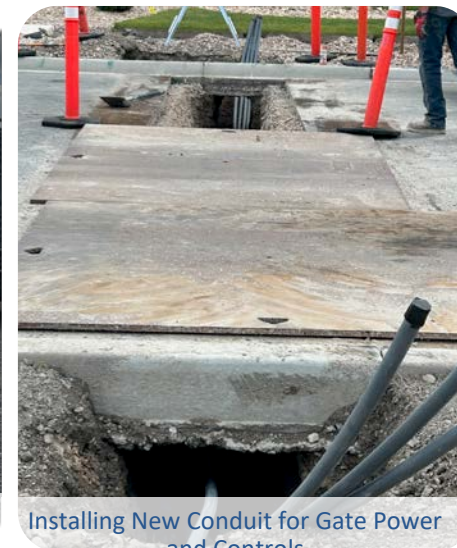
Installing Power and Control Conduit at Gate
