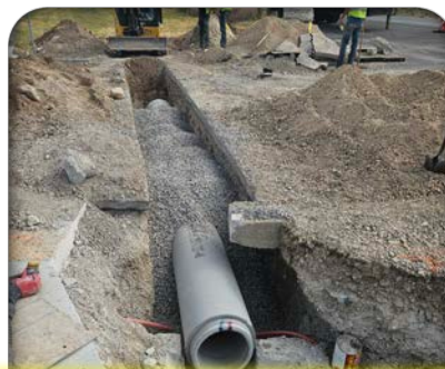
Supporting Contractor with new SD Pipe at McGregor
