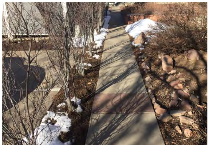
A narrow landscape strip between parking spaces and sidewalk provides a break in pavement and allows employment of simple drainage solutions. On the figure right, notice the flagstone mini bridge break in the concrete pavement where a mini ditch allows the water in the narrow landscape island to drain into the larger landscape island's open drainage system created by attractive mini ditches.
