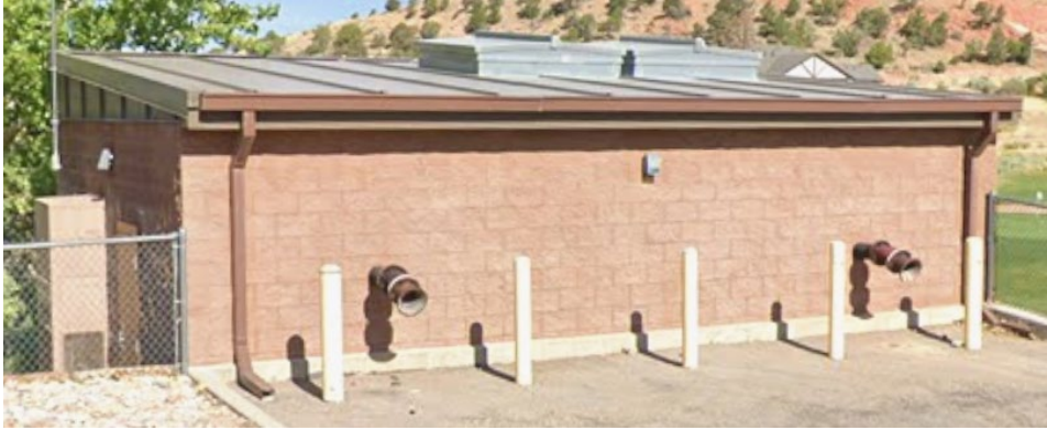
Golf Course Booster Pump Station (built in 2012)
