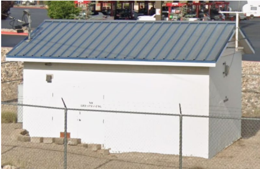
Square Mountain Pump Station (built in 1994)
