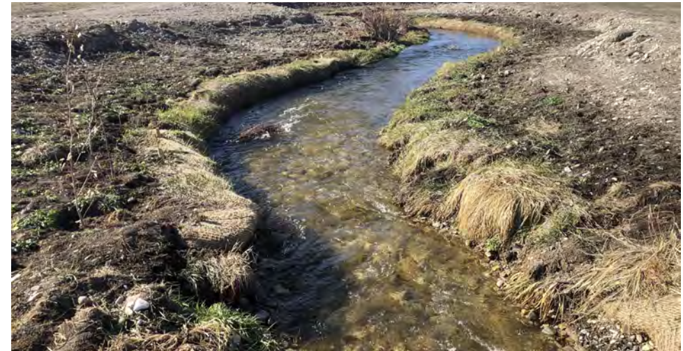
GROUND LEVEL VIEW OF SIDE CHANNEL AND RIPARIAN EDGE PROTECTION.
