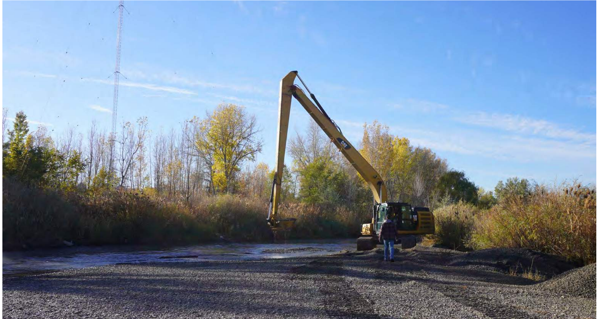
VIEW OF ONGOING RIVERINE MAINTENANCE AND EXCAVATION.
