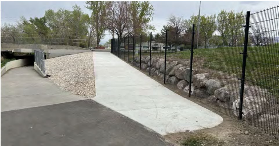
GROUND LEVEL VIEW OF CONSTRUCTED TRAIL LINK FACING 3300 S.
