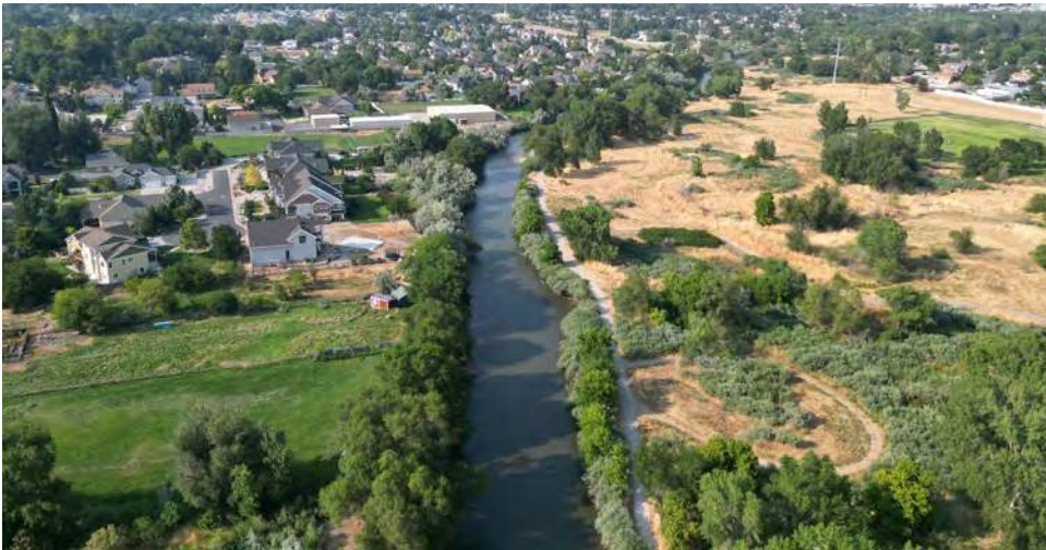
OVERLY STRAIGHTENED SECTION OF JORDAN RIVER NEAR 5400 S.
