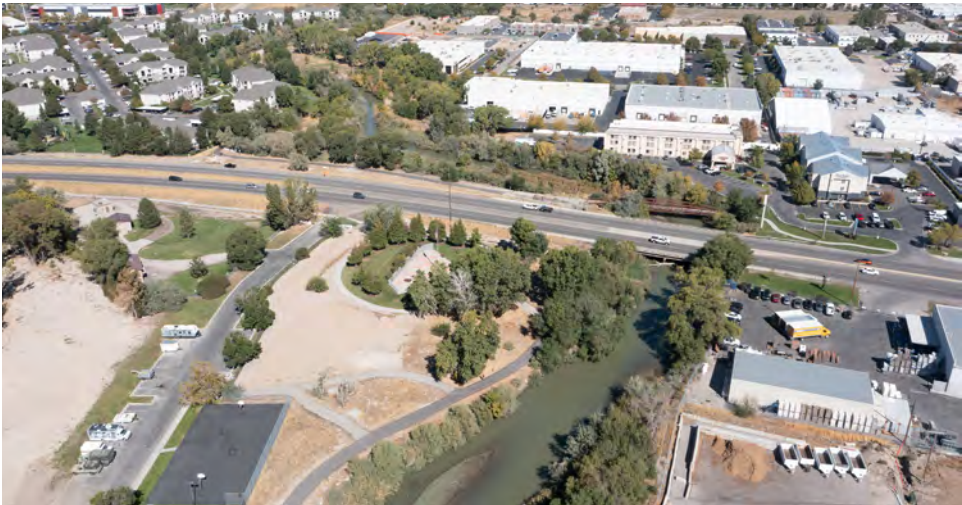
AERIAL VIEW OF PROPOSED ACCESS AND PARKING AREA LOOKING NORTH TOWARDS W TAYLORSVILLE EXPY
