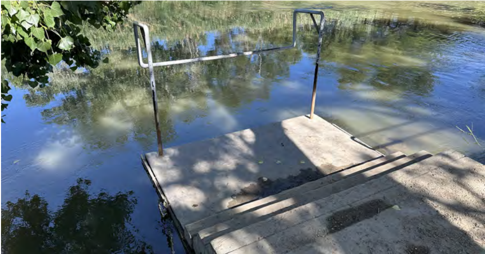
EXISTING BOAT LAUNCH AND RIVER ACCESS ACROSS FROM MILL RACE PARK IN MURRAY IS NOT ADA ACCESSIBLE.
