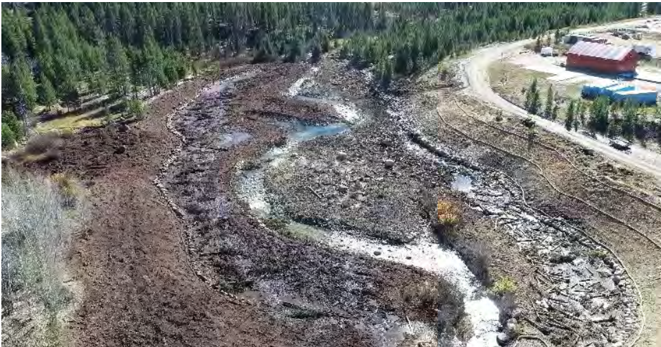
CHANNEL REALIGNMENT AND FLOODPLAIN CREATION IMMEDIATELY AFTER CONSTRUCTION; EAST FORK SOUTH FORK SALMON RIVER, ID
