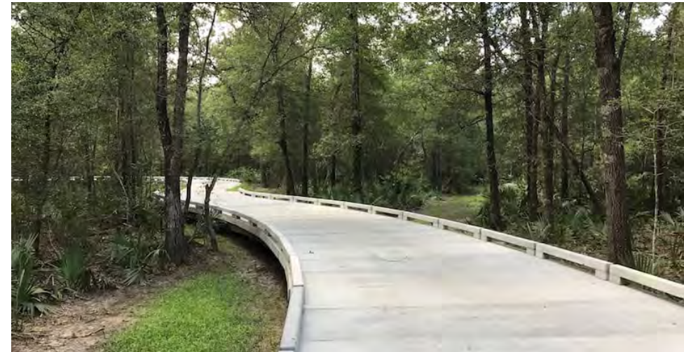
CONCRETE ELEVATED BOARDWALK AT HALLS BAYOU IN HOUSTON, TEXAS.
