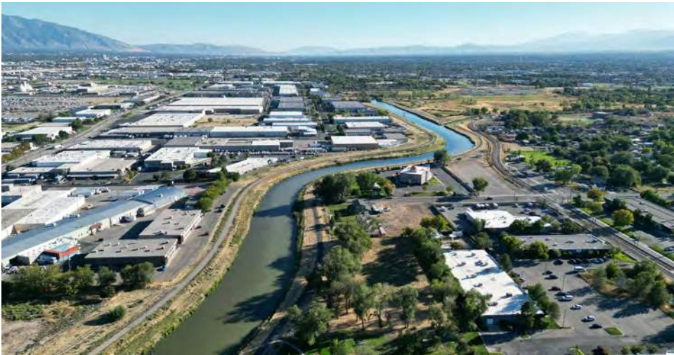
AERIAL VIEW OF THE JORDAN RIVER AND THE WIDE RANGE OF CONTEXTS—INCLUDING INDUSTRIAL, RESIDENTIAL, COMMERCIAL, AND ROADWAY—LINE THE CORRIDOR.
