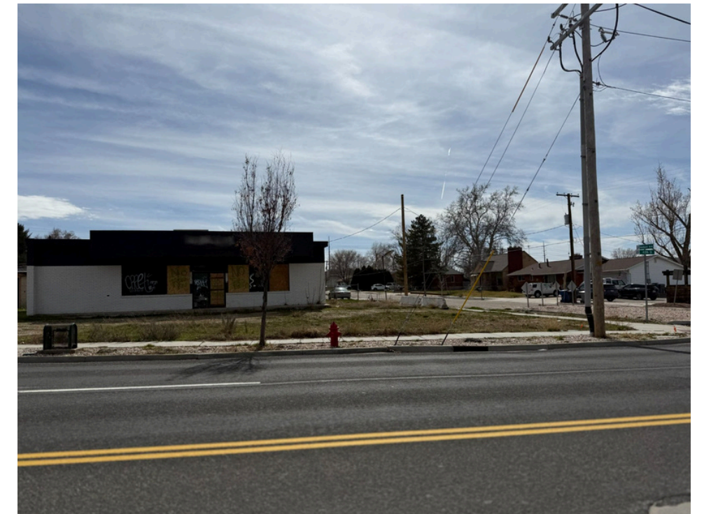
Example of a building in need of façade improvements Source: google.com
