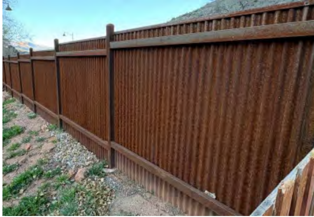
Figure 2. Example of proposed corrugated, rusted metal panels
