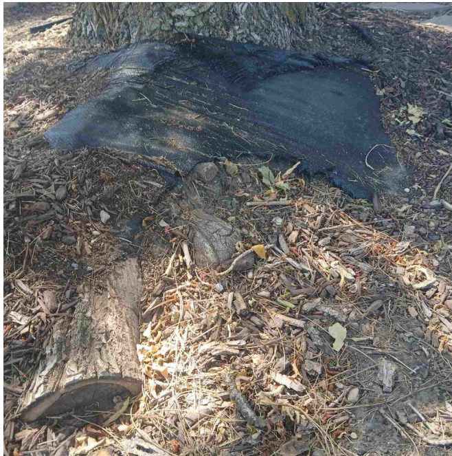
Photo 12. Tree 8. Root collar. Landscape fabric covers the root zone and obscures the collar. Cut root ends are exposed at the edge of the fabric in the foreground, showing the large diameter root cutting described in the Observations.
