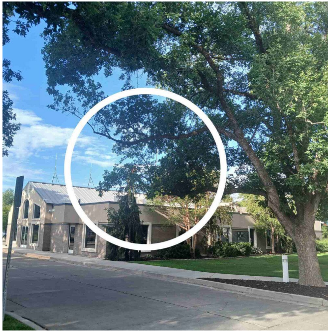
Photo 3. Tree 3. Tree 3 in relation to the existing municipal hall. Ringed: an overextended limb which should be reduction pruned.
