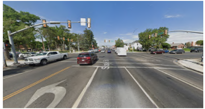
Signalized Intersection at State Street and 100 East
