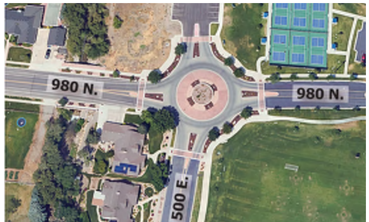
Roundabout at 980 N. and 500 E.
