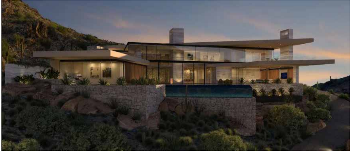
chimneys punctuate the dramatic horizontal roof overhangs
