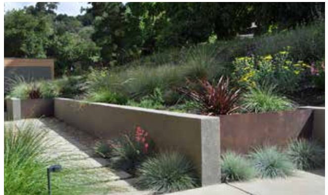
retaining wall composition with mixed materials
