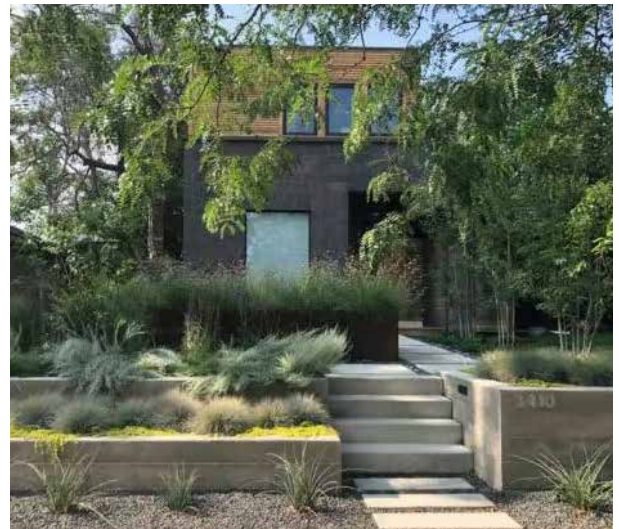
front steps are integrated with retaining walls
