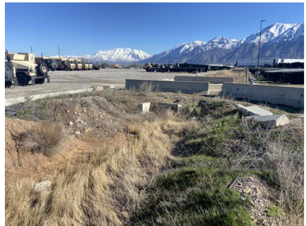
2' W x 5' H Concrete Box Culvert (most upstream)
