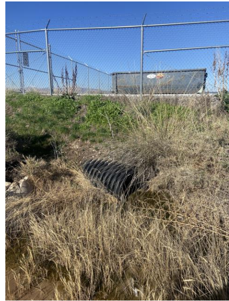
27-inch corrugated HDPE (Downstream side)
