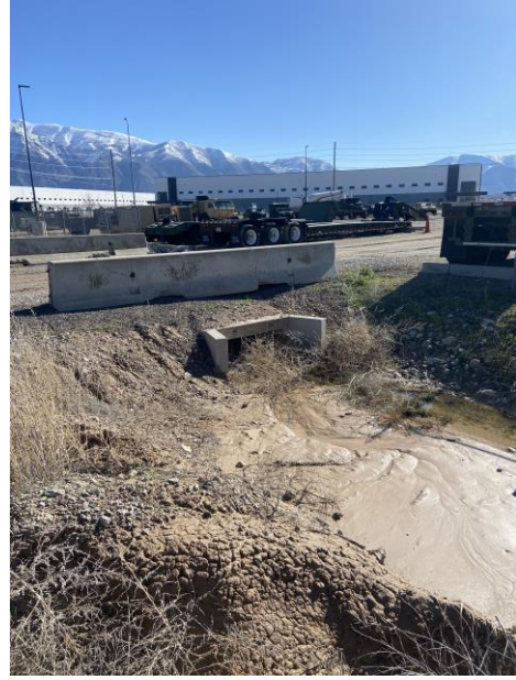
2' W x 5' H Concrete Box Culvert (most downstream)
