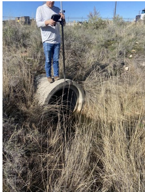
36-inch RCP (Downstream side)
