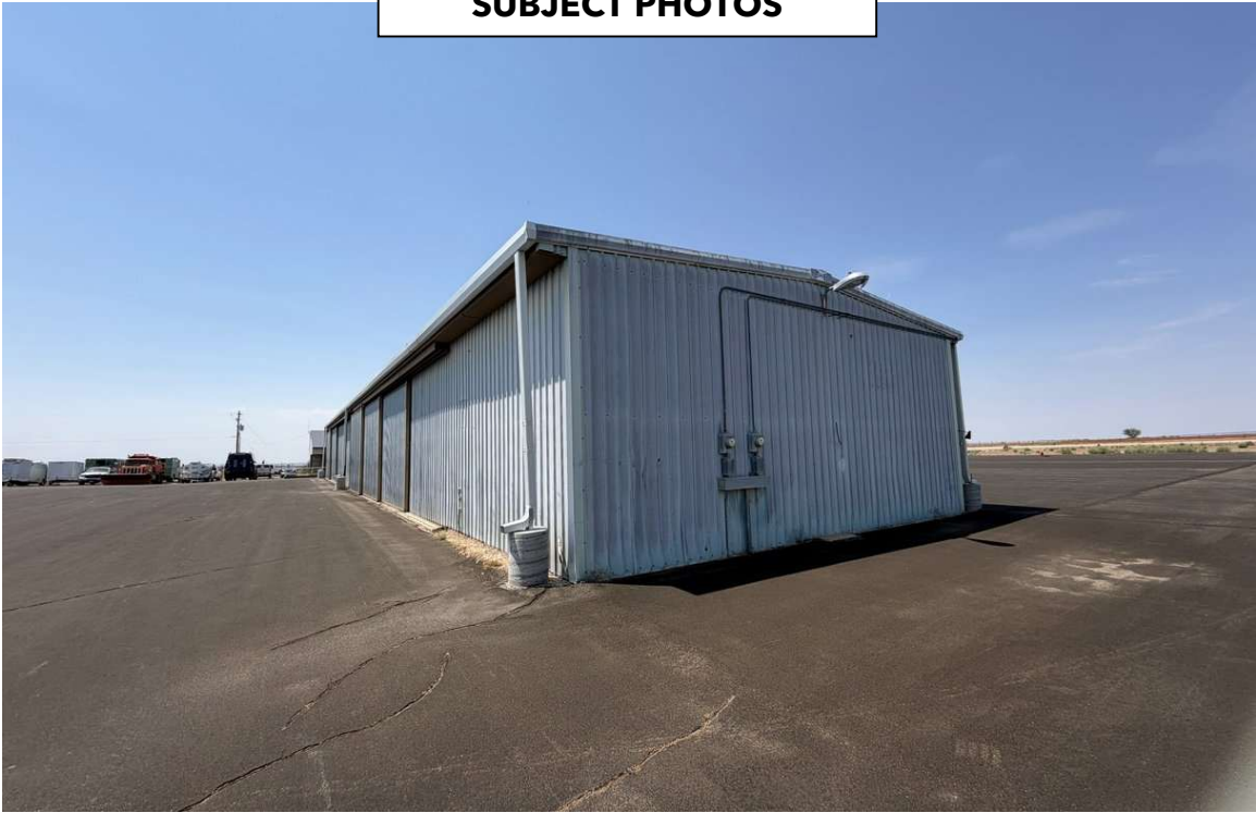
EXTERIOR OF SOUTH BUILDING
