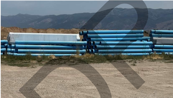
Water Pipe Stockpile (View: Northeast)
