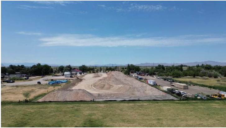
Site Overview (View: West)
