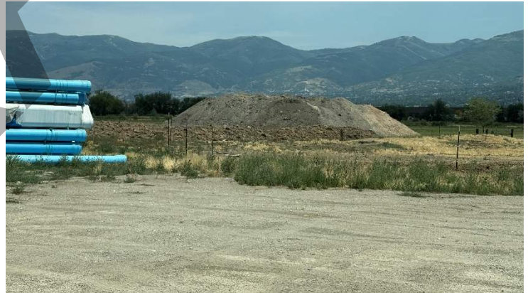
Onsite Material Stockpile (View: Northeast)
