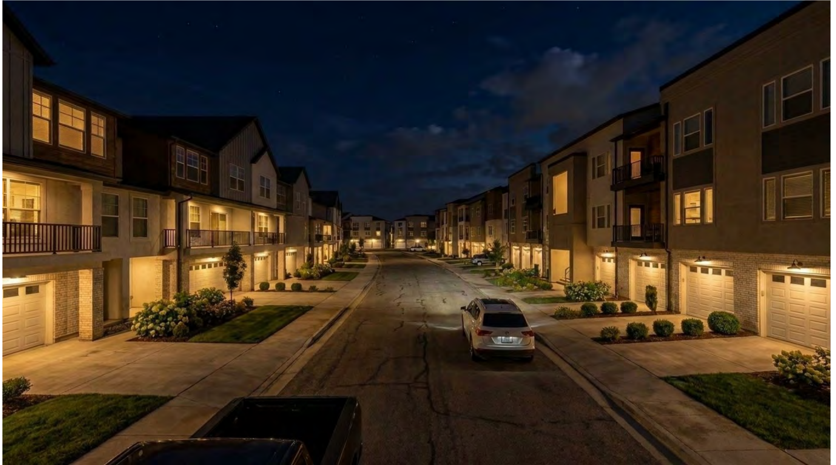
Project/ Street Lighting (Located on Buildings)
