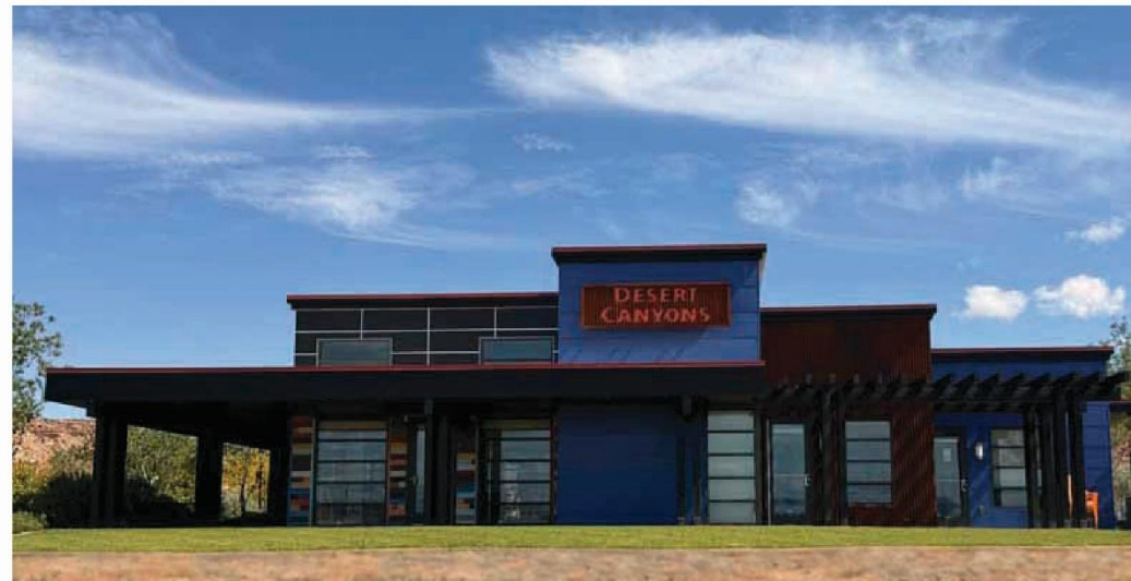
OFFICE BUILDING REAR ELEVATION
