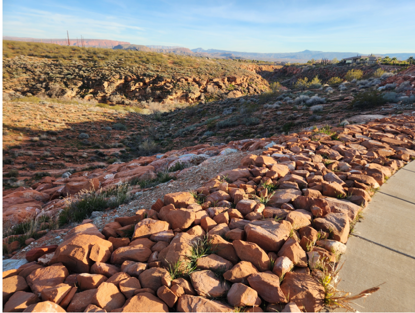
Looking Southeast from 590 West Street at Fill slope
