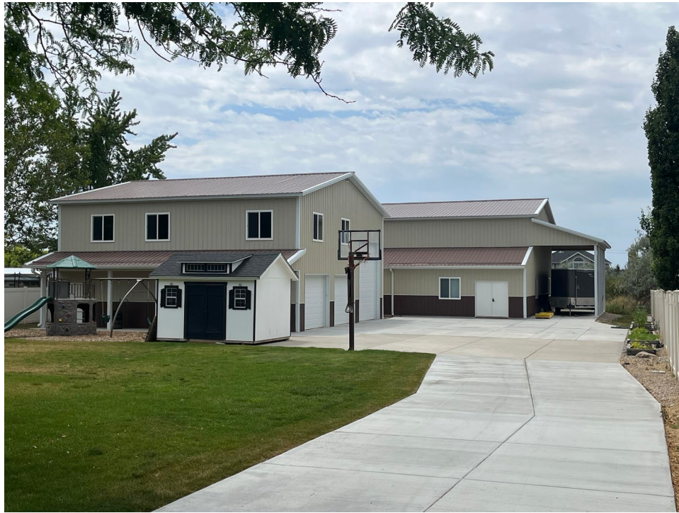
Two-story metal accessory building, tan siding with dark brown wainscoting, standing seam roof. Comparable scale to the Racker building, visible from the street.
