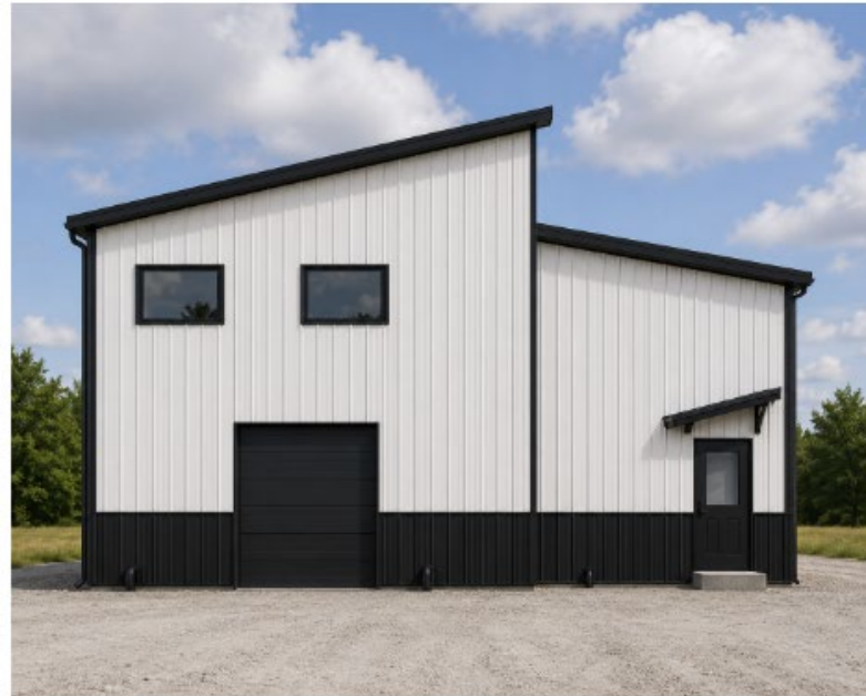
Front/corner elevation — white R-panel siding, black wainscoting, black standing seam roof and trim.
