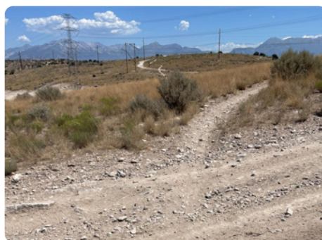
ObjID 68, Backspace: Road crossing with no signage.
