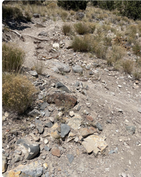
ObjID 25, Flintstone: Switchback Slope is too steep
