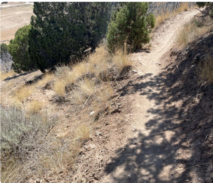
ObjID 59, Cougar Tracks: Trail is peeling away, skidded trail cuts off to the left.
