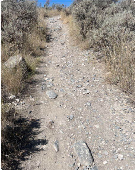
ObjID 6, Connector: Slope exceeds 10% for over 100 feet. Slope does not match difficulty.
