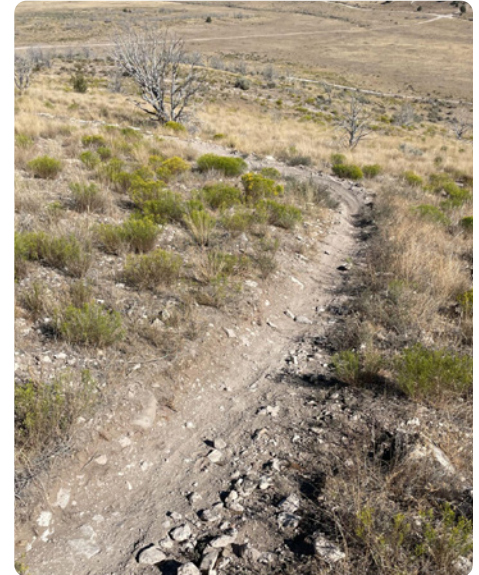
ObjID 86, Eastwood: Slope exceeds max recommendation.
