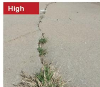
Figure 2 - Cracking
