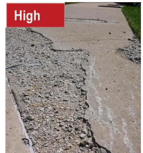
Figure 3- Spalling
