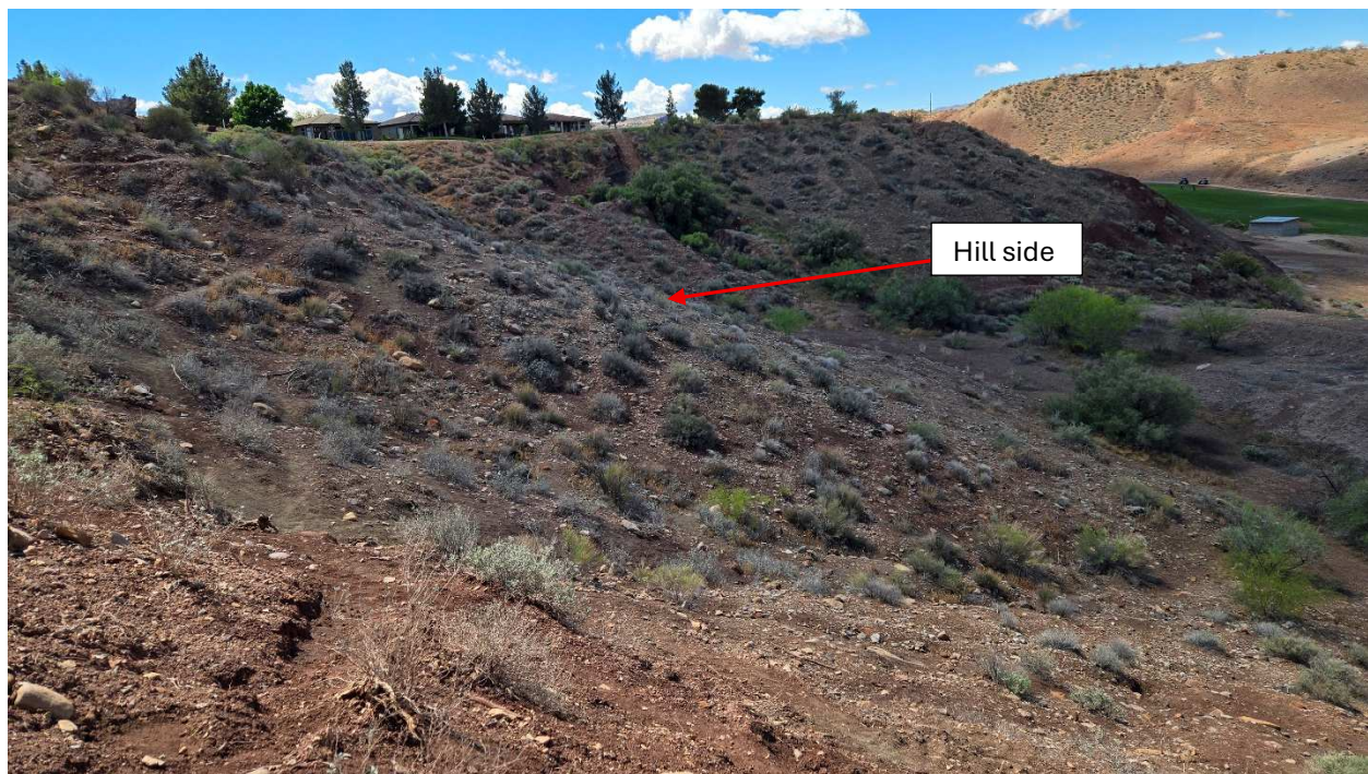
Photo 4: View of the hillside along the east side of the subdivision. Slopes are approximately 2\frac{1}{2}:1 (Horizontal:vertical) or flatter.
