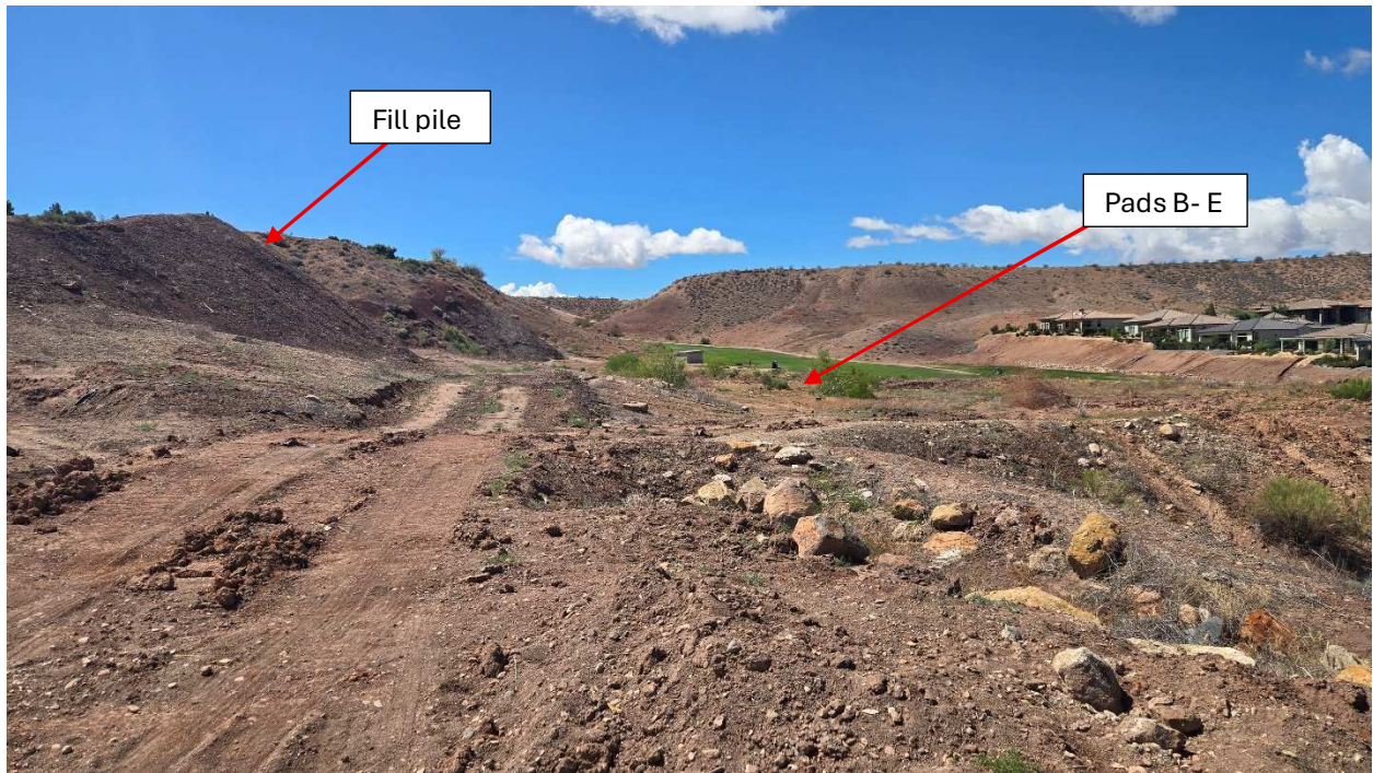
Photo 1: View of the location of the proposed drive looking south.
