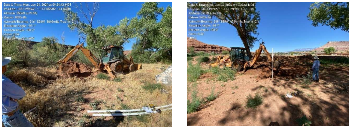
Figure 7: Field installation of piezometer casings on June 24, 2024.
