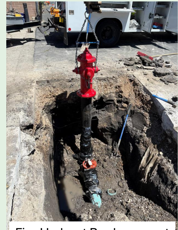
Fire Hydrant Replacement 850 S Industrial Area
