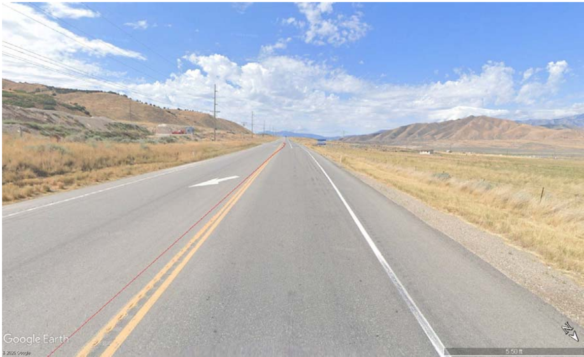
Looking South from North of the Intersection
