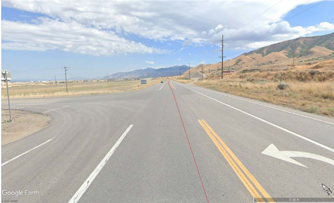
Looking North AT the Intersection
