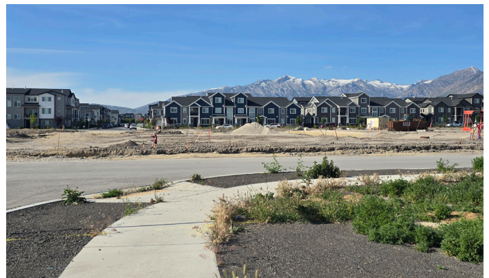
Multi-Family Residential & Construction to the North
