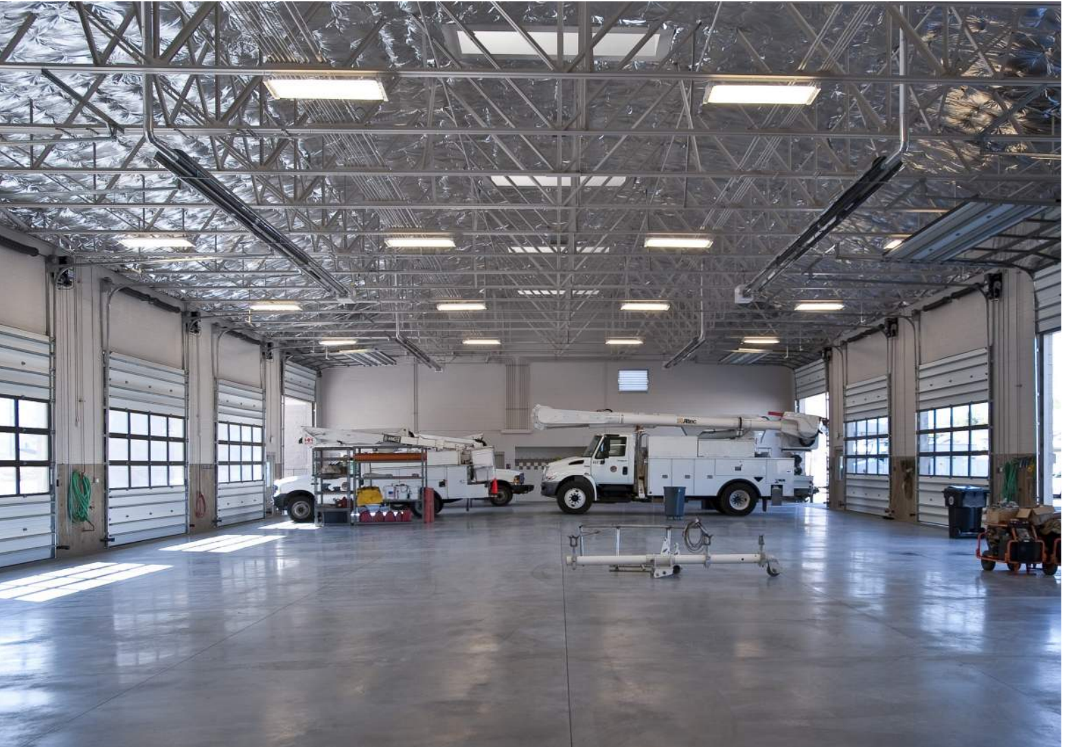
Springville C Electric Operations Buildi
