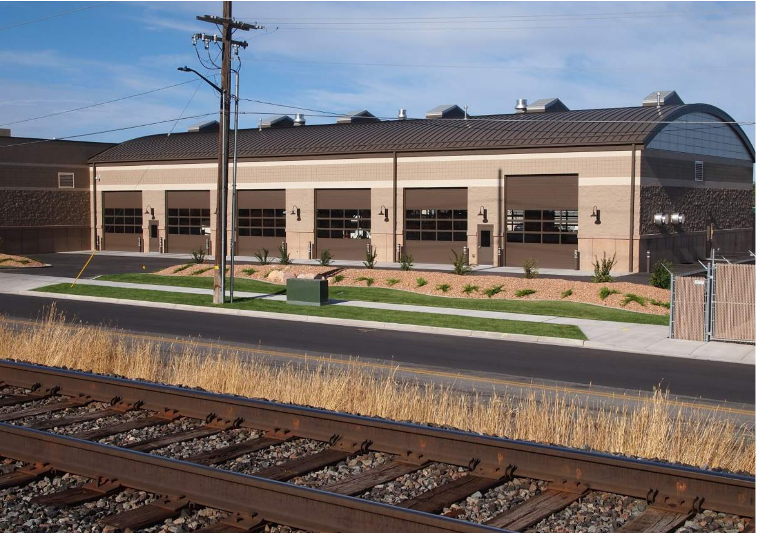
Springville C Electric Operations Buildi
