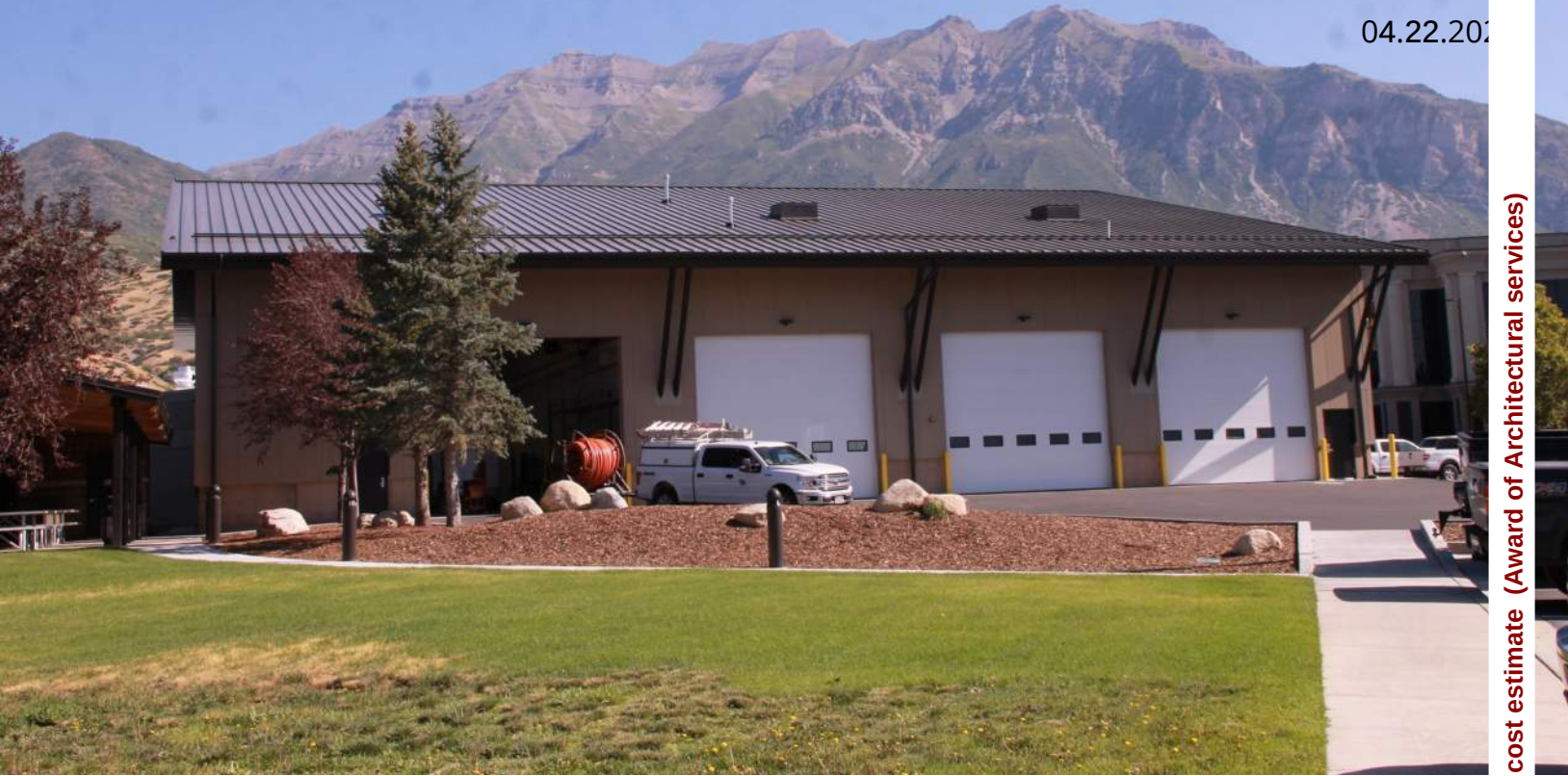
Central Utah Water Conservancy District Operations Building
