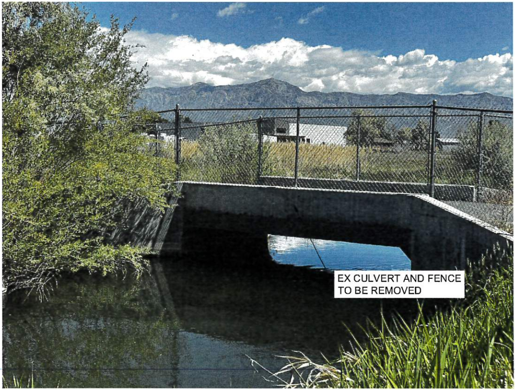
WEST SIDE OF TRAIL LOOKING EAST
