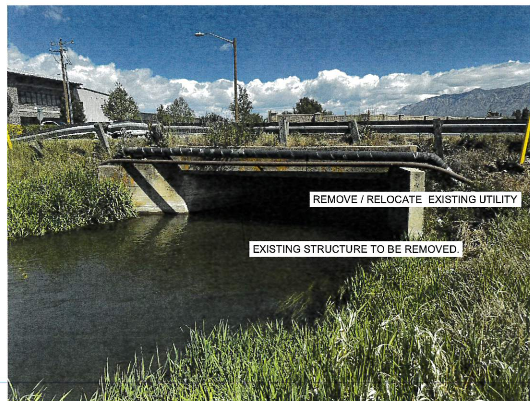
WEST SIDE OF TRAIL LOOKING EAST
