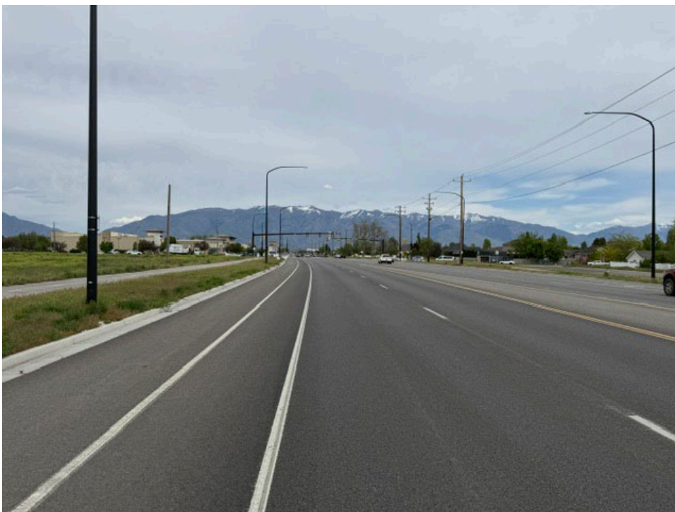
Looking easterly along the subject surplus parcel frontage on Antelope Drive.
