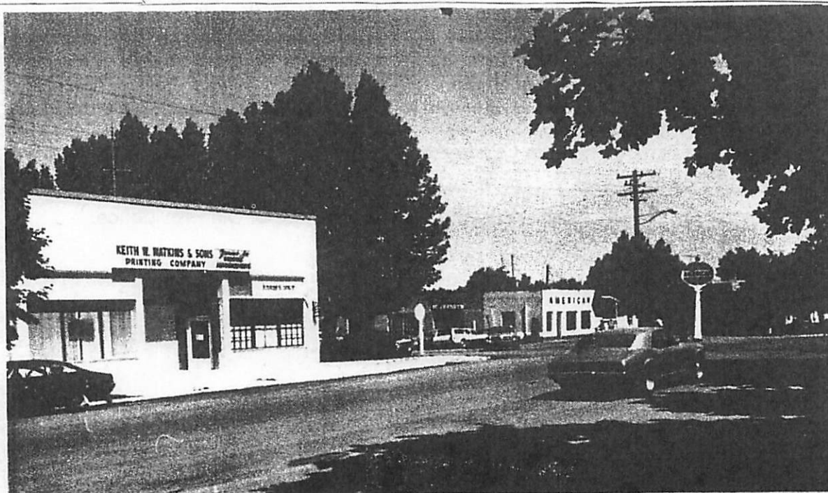
View of Main Street looking north.
