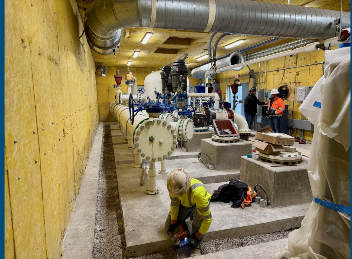
Floor Drain Installation
